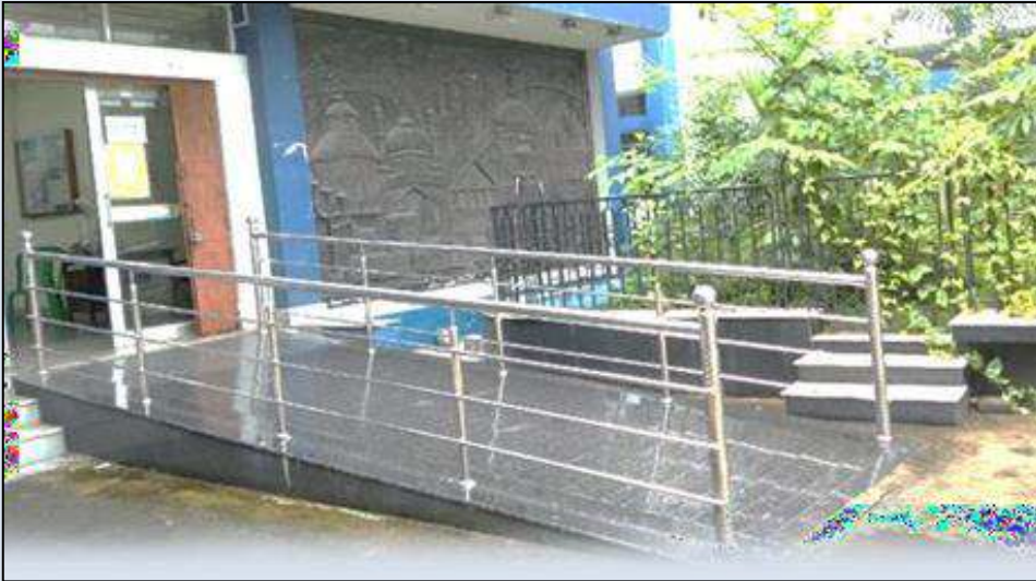
Ramp at the Entry Gate
